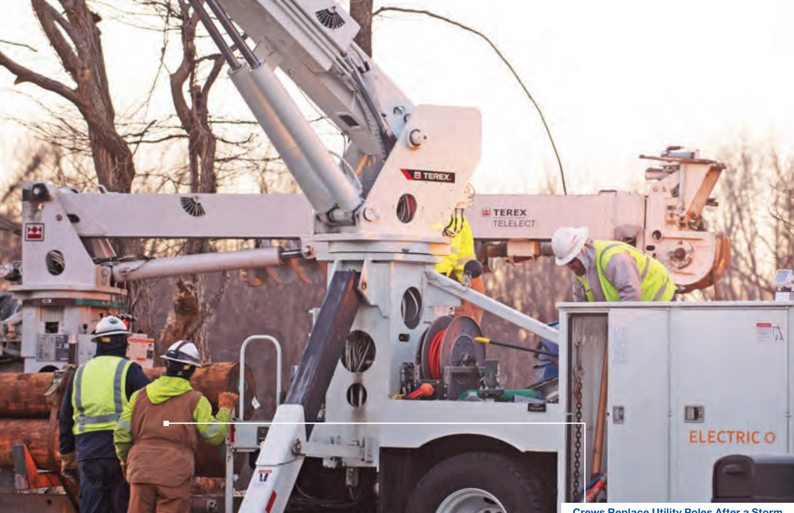
Crews Replace Utility Poles After a Storm
