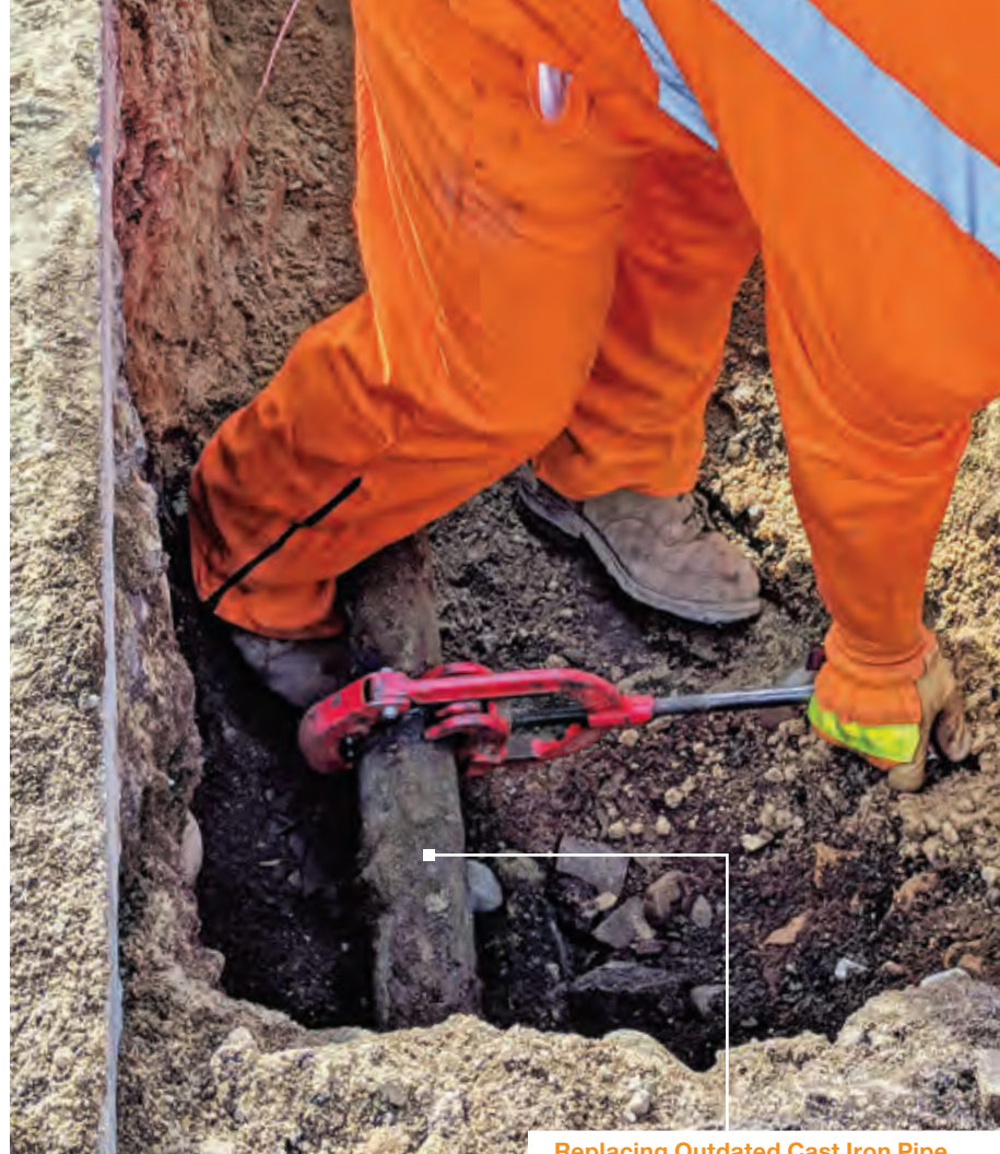
Replacing Outdated Cast Iron Pipe
