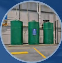
On-site tanks to collect, treat and store rainwater for use in washing trucks, and low-flow toilets and water fixtures — combined, these will save an estimated 60,000 gallons of water annually
